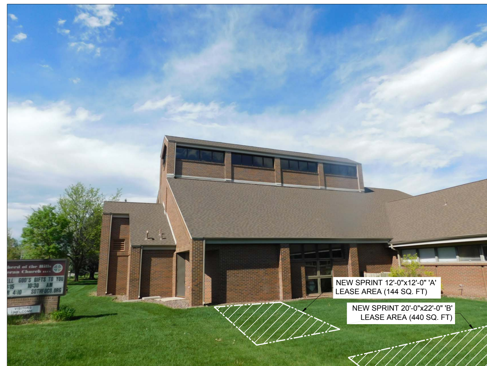
VIEW OF NEW LEASE AREA (LOOKING NORTHEAST)
