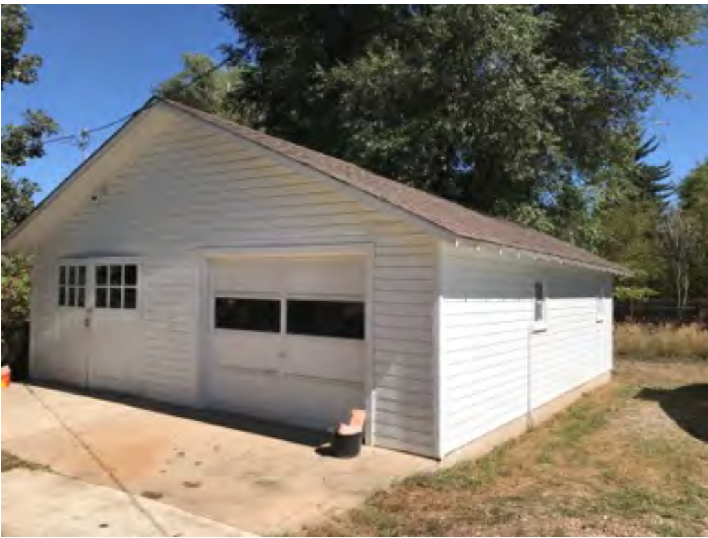
Above: view of existing garage west and south sides.
