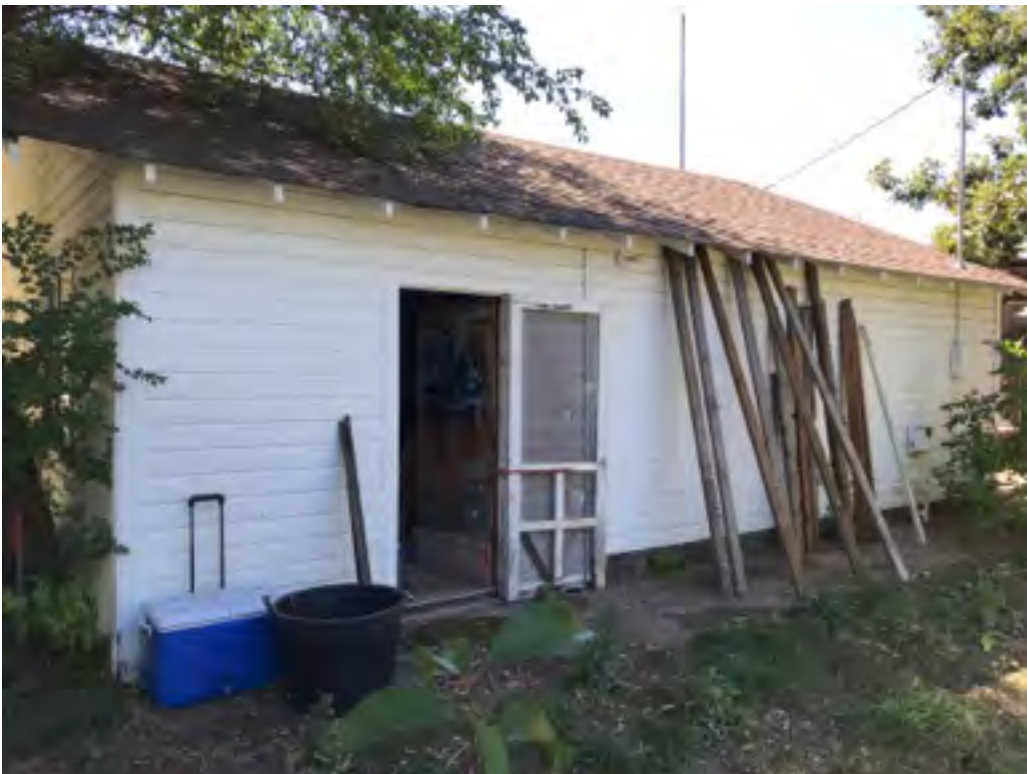
Above: view of existing garage east and north sides.
