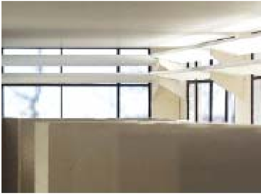
Dual light shelves reflect light across the ceiling for more balanced daylighting
