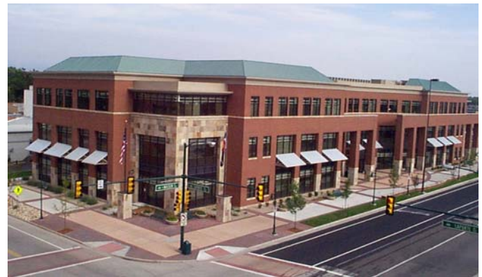
215 North Mason Office Building – Exterior shading helps reduce direct sun of the first floor.
