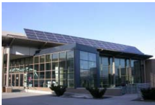
Fig. 6: Performing Arts Center 10 kW Solar Array
