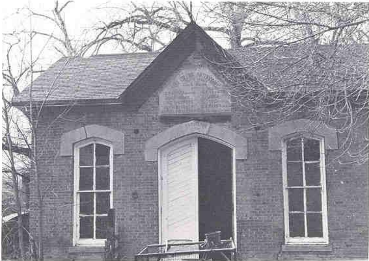
Original waterworks building constructed in 1882.
