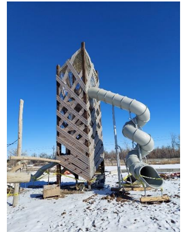
Play structure installed at Dovetail Park.
