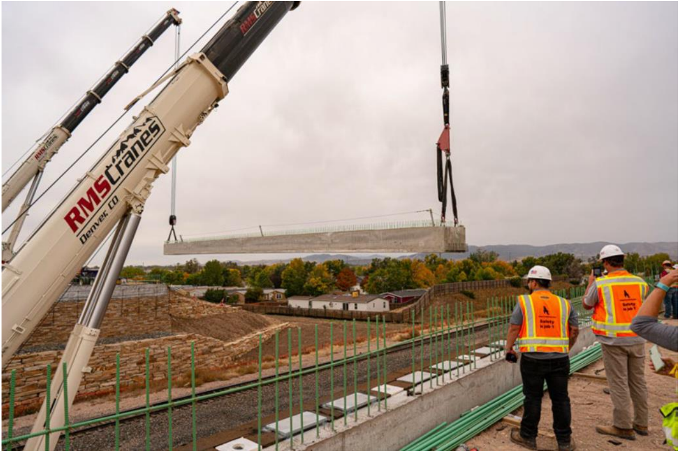
Construction of the Vine and Lemay overpass
