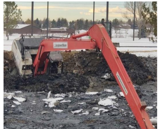
Pond dredging at Southridge Golf Course
