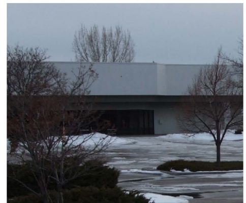
Large vacancies such as the former Walmart provide opportunities for new housing and mixed-use development in Midtown.
