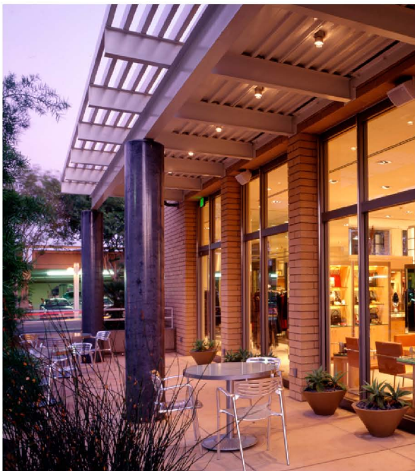
Weather conditions will be addressed to maintain an acceptable level of customer comfort in outdoor areas.
