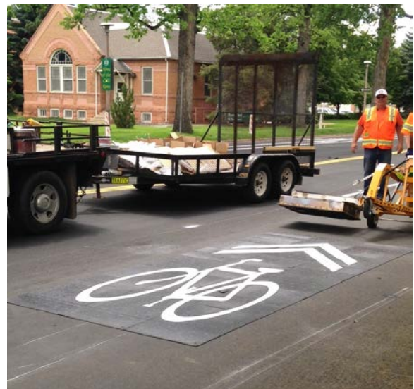
Application of a sharrow marking on Laurel Street
