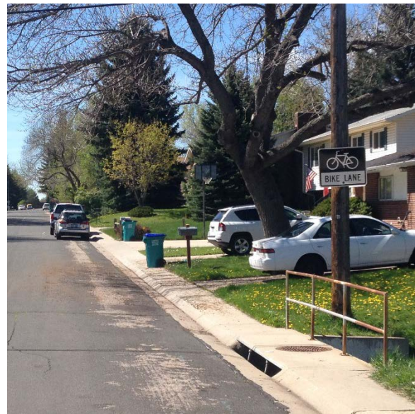
Missing pavement markings or incorrect sign
