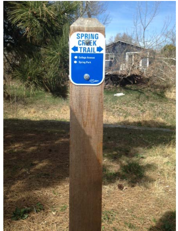
Trail confirmation signs are small, hard to read at bicycle speeds and text is often obstructed by mounting hardware.
