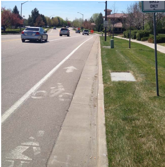
Worn pavement marking in need of maintenance
