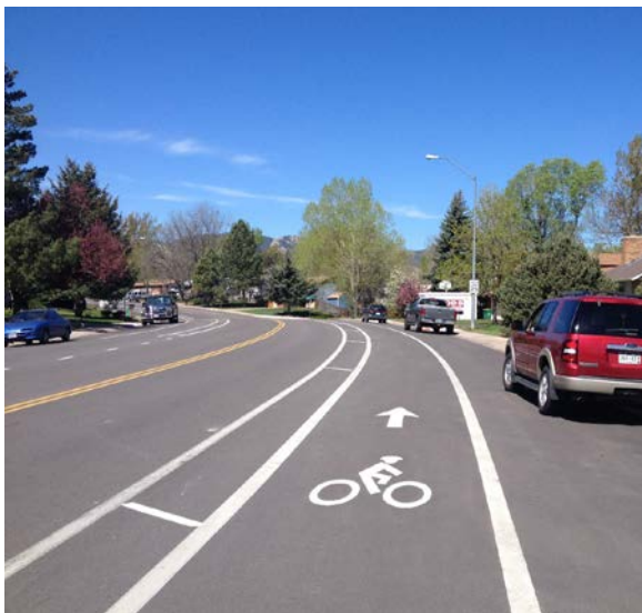
A new buffered bicycle lane on Stuart Street provides an enhanced facility and traffic calming for a local street
