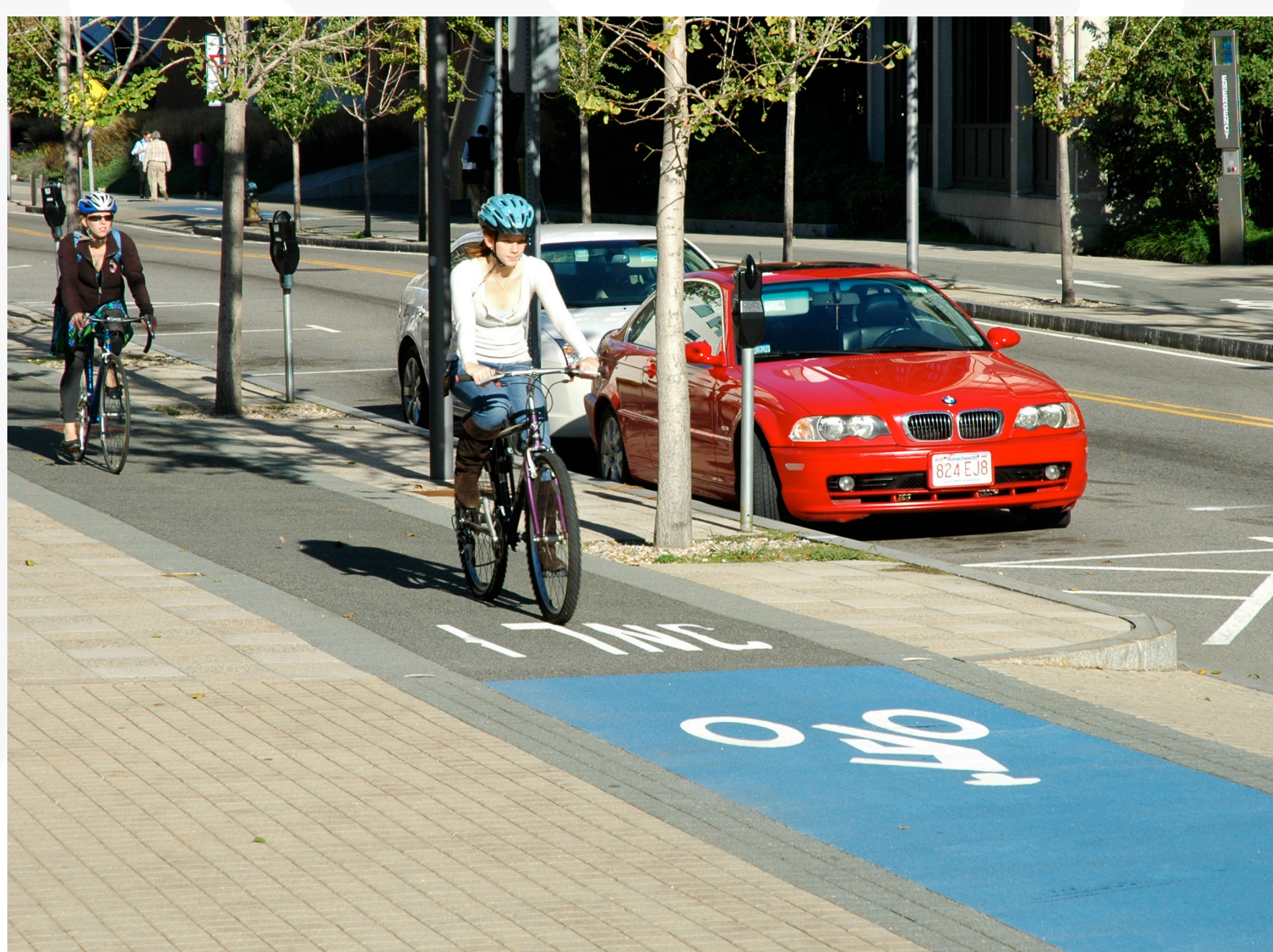
Colored driveway crossing Alerts users of conflicts
