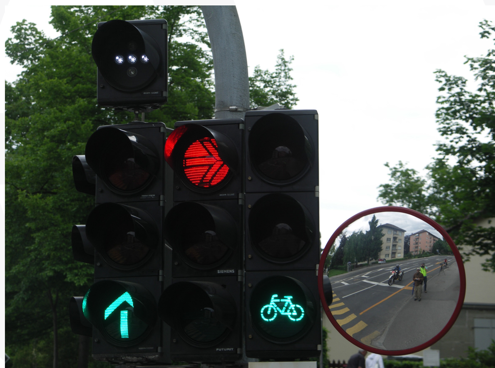
Bike signals Separates conflicts
