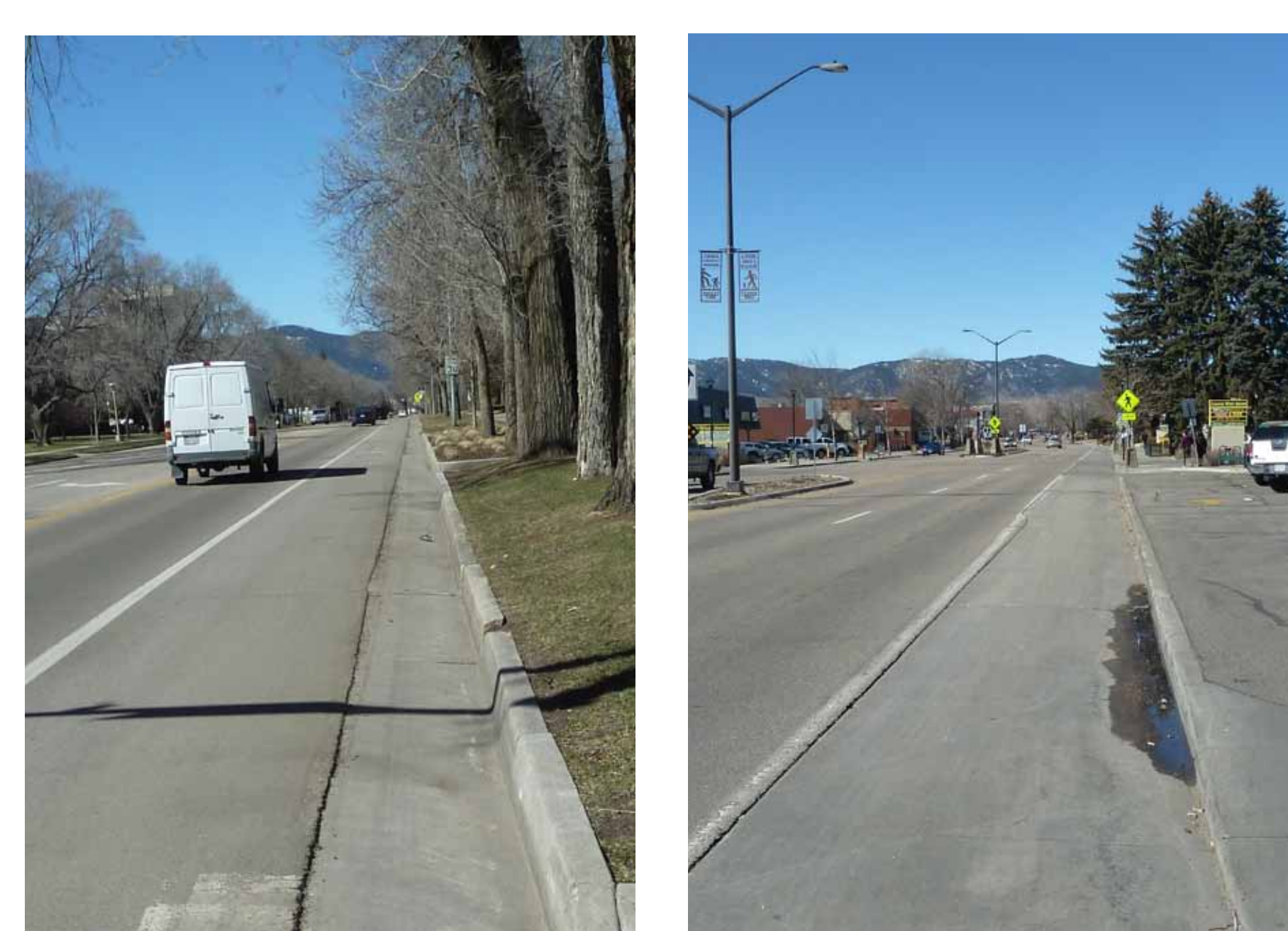
Unsafe gutter pan Safe gutter pan
