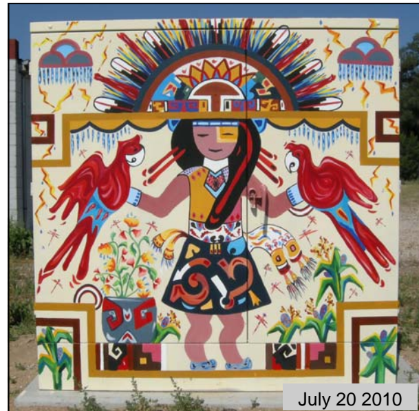
The completed cabinet: East Side
