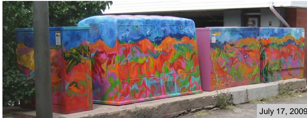
The completed group of cabinets with the 2009 mural second from left
