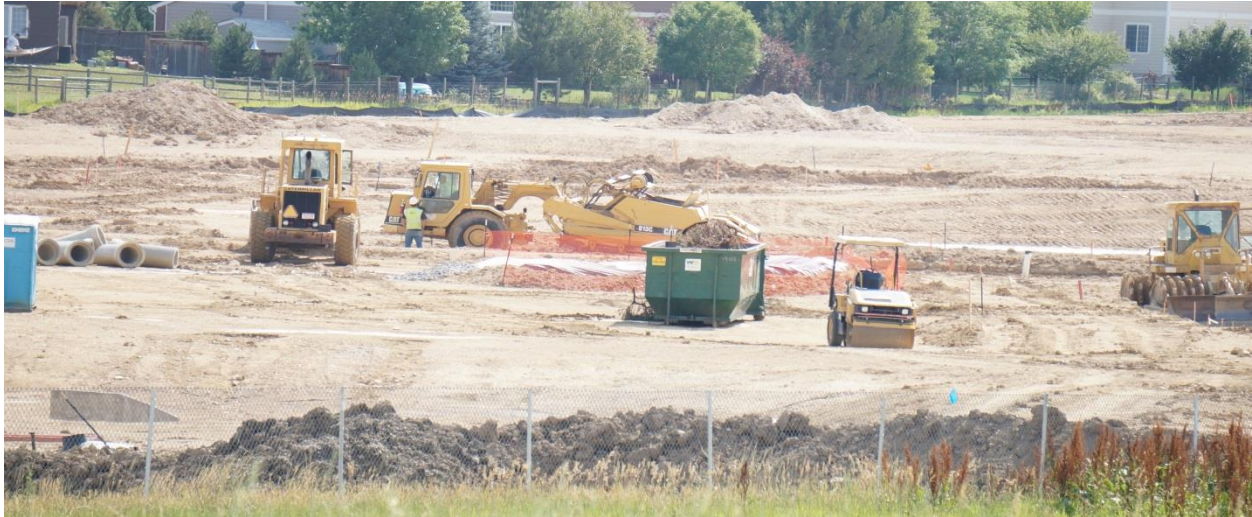
Above: This figure illustrates earthmoving, which is an activity that can generate dust.
