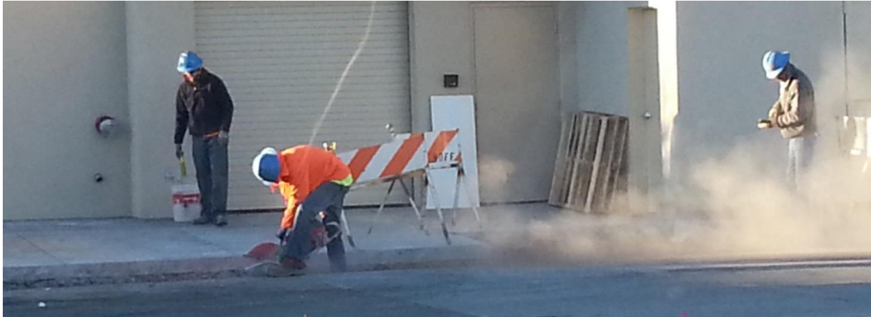
Above: This photo illustrates concrete cutting and how the activity can generate dust.
