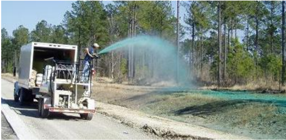
Left: This photo represents adding vegetation by hydroseeding, which is one measure to comply with the Manual.
