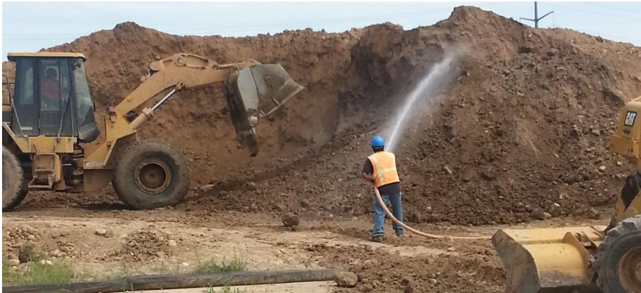
Above: This photo illustrates wet suppression, an additional best management practice for stockpiles.
