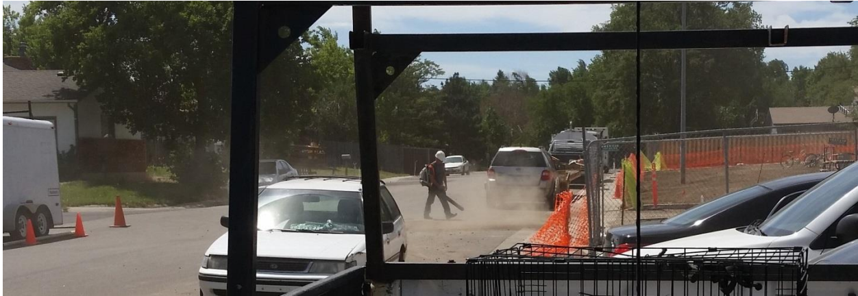
Above: This photo illustrates mechanical blowing without dust mitigation in place.
