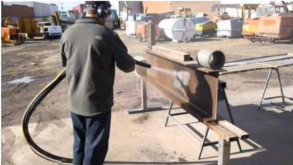
Above: This photo illustrates wet suppression blasting, an additional best management practice.
