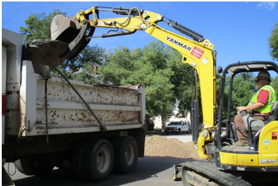
Above: This photo illustrates reducing drop height, a required best management practice.
