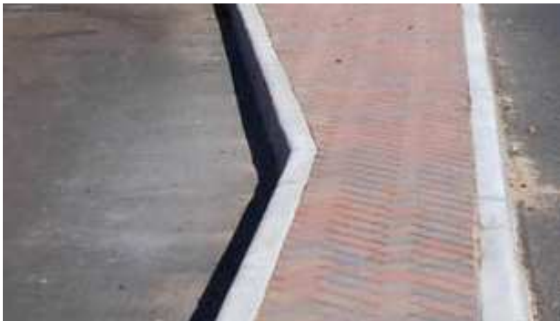
Rectangular pavers set in a herringbone pattern.
