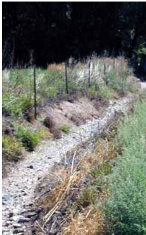
Additional planning and stormwater improvements will help reduce flooding potential in the area.
