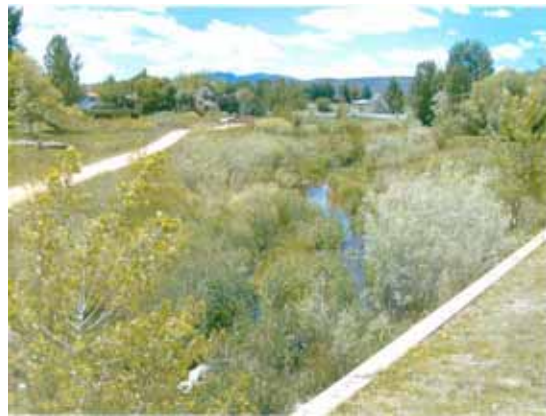
Restoration of Soldier Creek will provide trails and open space in addition to accomplishing drainage objectives.
