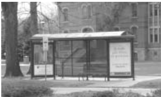
Bus shelters need to be improved, such as in this example.
