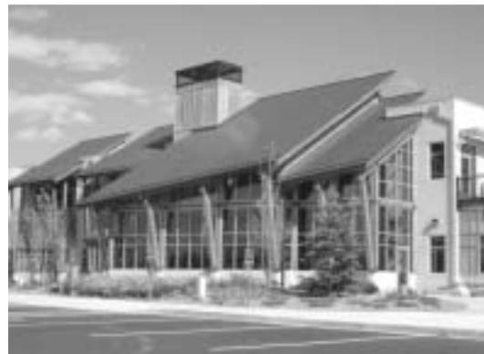
Newly-built In-Situ headquarters south of Buckingham.
