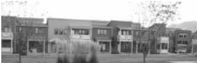
Live-work example - Steelyards project in Boulder, CO.
