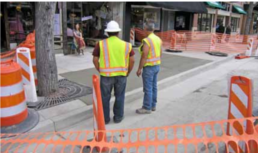
New sidewalk, curb, and gutter fitted in among older existing portions of sidewalk that were in good condition.
