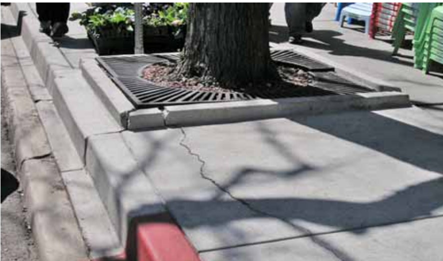
Example showing cracks and heaving in concrete sidewalk and tree grate curb.
