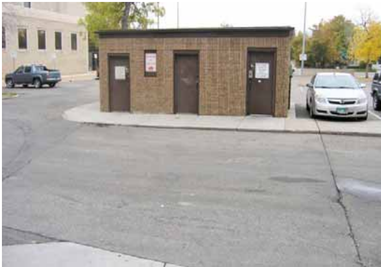
The existing public restroom.
