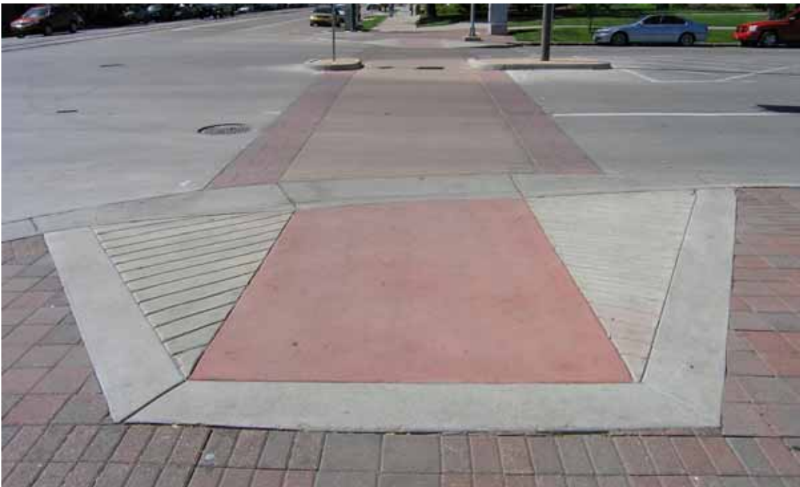
Example of an enhanced crosswalk with colored, textured paving, a median refuge, and corner plaza pavers.
