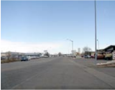
Link Lane at SH 14 looking north, illustrating the need for upgraded urban services.
