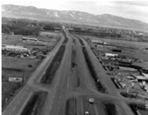
1968 aerial showing a 12 year-old SH 14 bypass.
