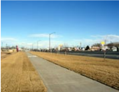
East Mulberry Street at Lemay Avenue streetscape improvements.
