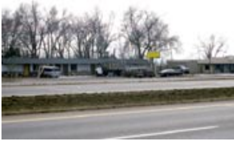
View of the South Frontage Road, illustrating the need for urban street standards.
