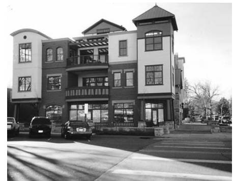
A transitional area mixed-use development with ground floor and upper floor residences.
