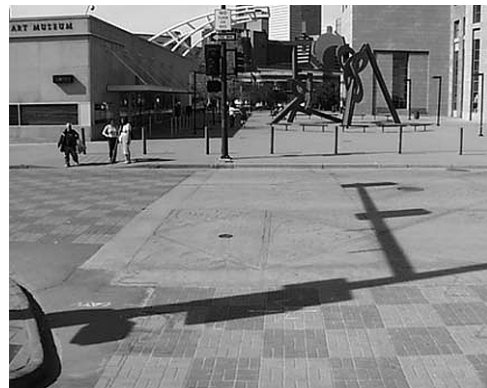
Intersection treatment using colored pavement.
