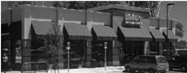
New building reviewed under the Land Use Code, The projecting entrance area demonstrates these standards.
