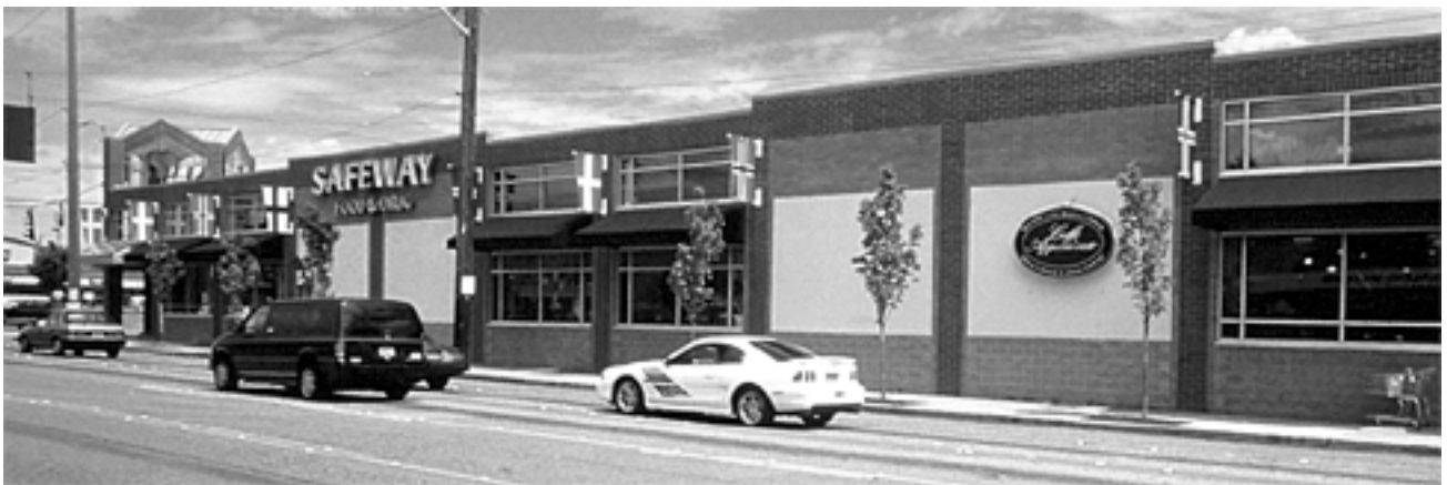
Supermarket site redeveloped to take its place along the street and allow updated development on an outdated site. Fort Collins standards would call for a little more room along the street edge, with a little more landscaping.
