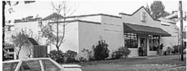
Massing variation in a modest neighborhood commercial building. (Caused by the sloping ground in this case).
