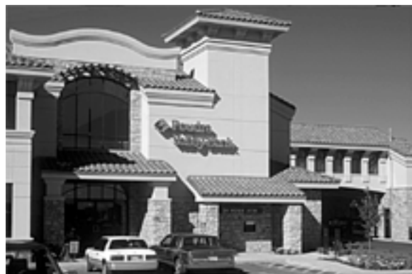
2 stories including occupied space above drive-thru.
