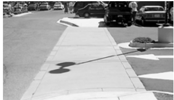
Nicely scored, tinted, lightly textured concrete.
