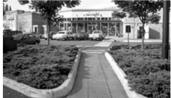
Walkway island with no ramps up and down.
