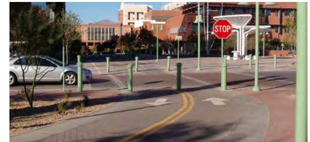
Colored concrete pavers increase the visibility of a shared-use path crossing a roadway in Tucson, Arizona.
