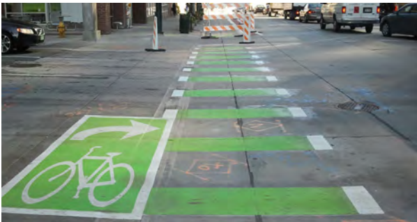
Intersection crossing markings in Denver, Colorado raise awareness for both bicyclists and motorists to potential conflict areas.
