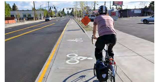
Pavement markings at this driveway crossing on the Cully Street Cycle Track in Portland, Oregon notify cyclists and drivers of a potential conflict area.
