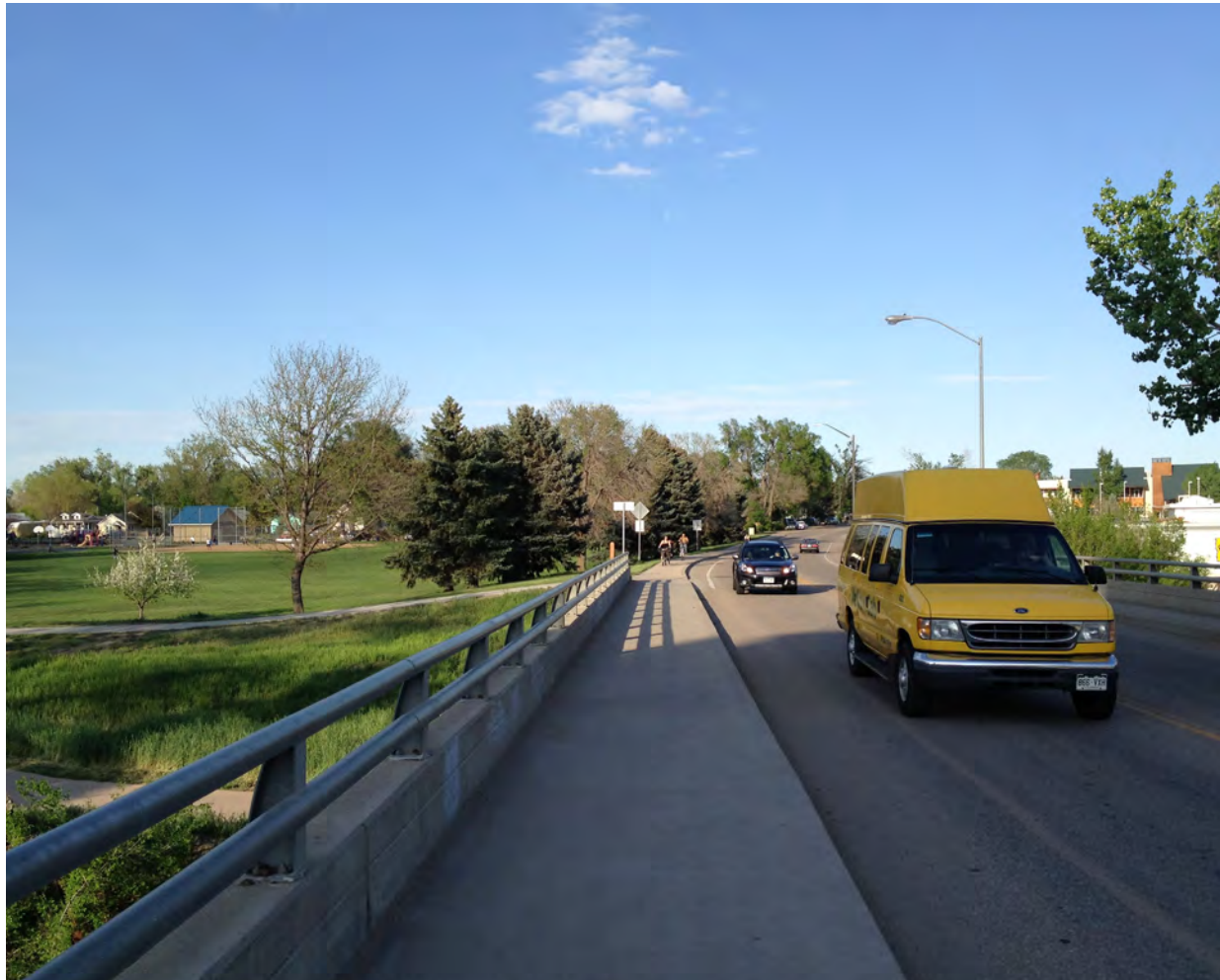
Lincoln Corridor Bridge
