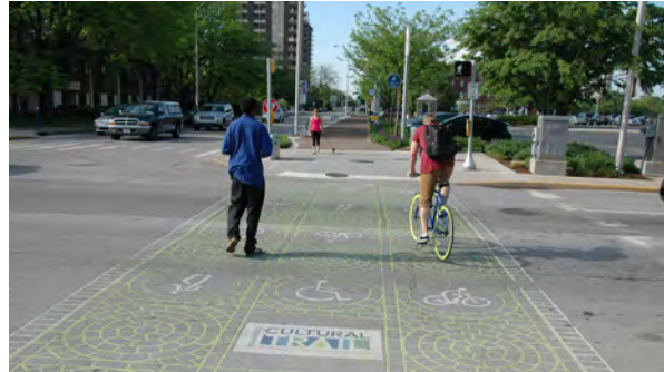
A crosswalk in Indianapolis, Indiana provides dedicated space for users of a Share-Use Path at a roadway crossing.
