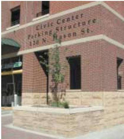
Mason Street serves multiple transportation modes, such as automobiles at the recently completed Civic Center Parking Structure
