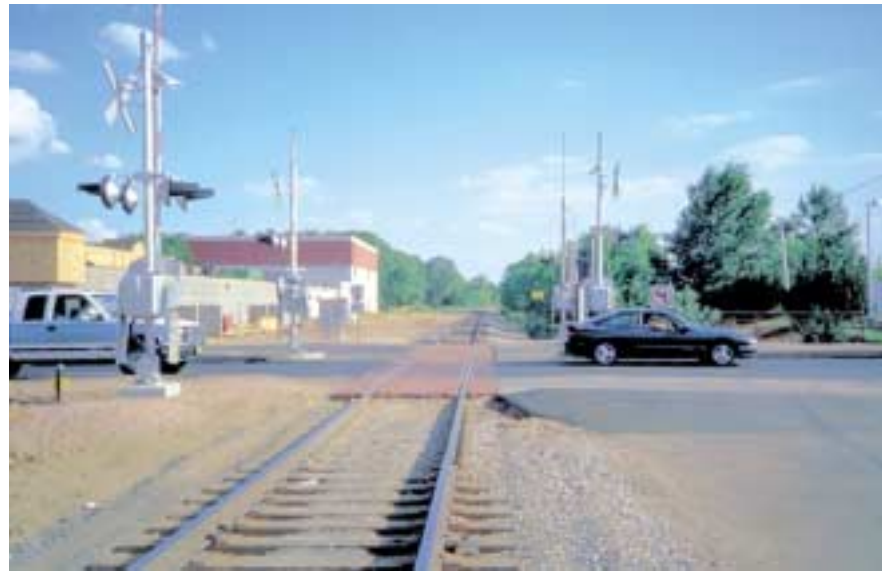
Development abuts BNSF Railway right-of-way.
