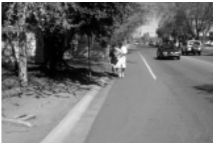
Stretch of Plum lacking sidewalk.
