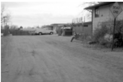
Existing 1/2-block segment of Scott St. on south side of Plum. R.O.W. is 20’ wide, surface is unimproved except for gravel.
